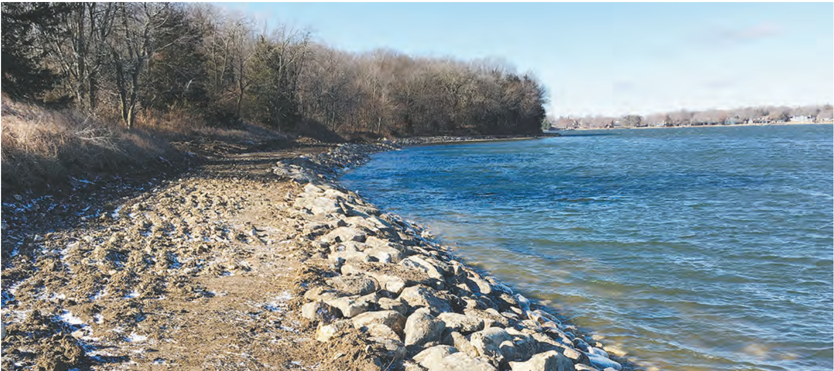
This shows the progress being made to repair rip rap along the south shore of Lake Panorama's main basin. The work began at the ski team dock and will continue west all the way to the dam.
