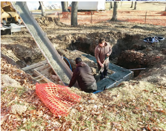
Good fall weather allowed work to begin on new bathrooms at both Shady and Sunset beaches. Here Kane Powell and one of his employees pour concrete footings Nov. 29 for the new bathroom at Shady Beach.
