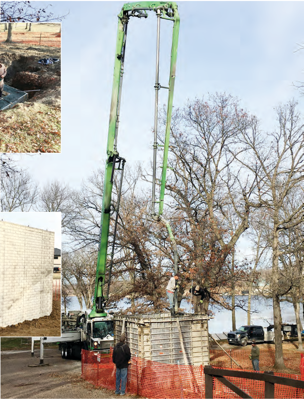
The beach bathrooms are identical in size and design, which includes poured concrete walls and roofs made with wooden trusses and corrugated steel sheeting. The concrete walls were poured at both locations Dec. 1. This photo shows the work being done at Shady Beach.
