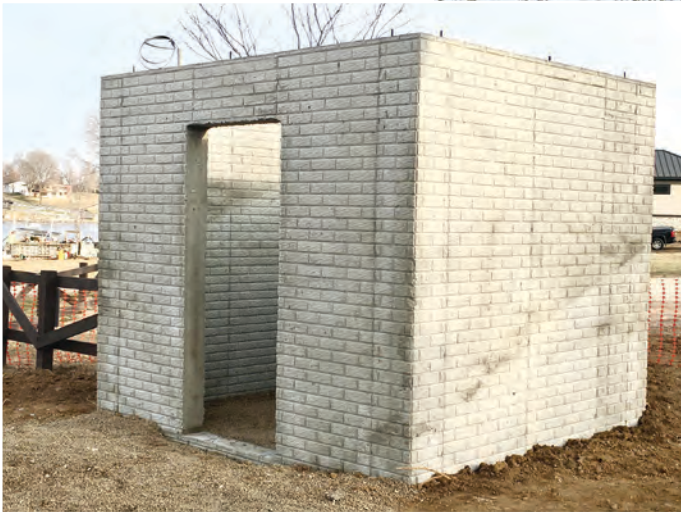
This structure at Sunset Beach shows the 8-foot by 10-foot size of these new bathrooms, which will be unisex, include one stool and sink, and be large enough to comply with federal regulations for handicap accessibility.
