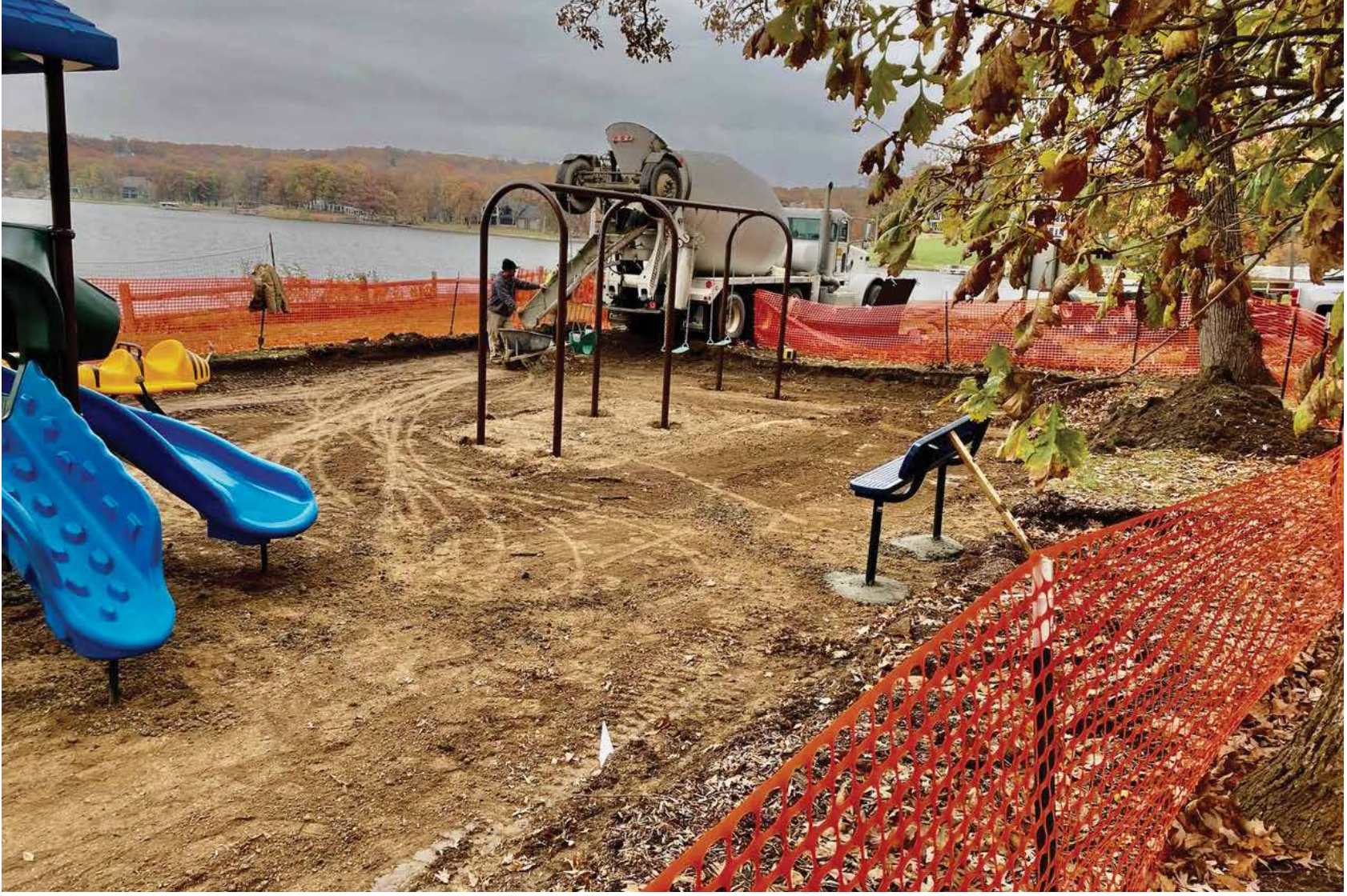
Installation by Boland Recreation included pouring concrete footings to secure a bench, three swings, spring rider and the playset.
