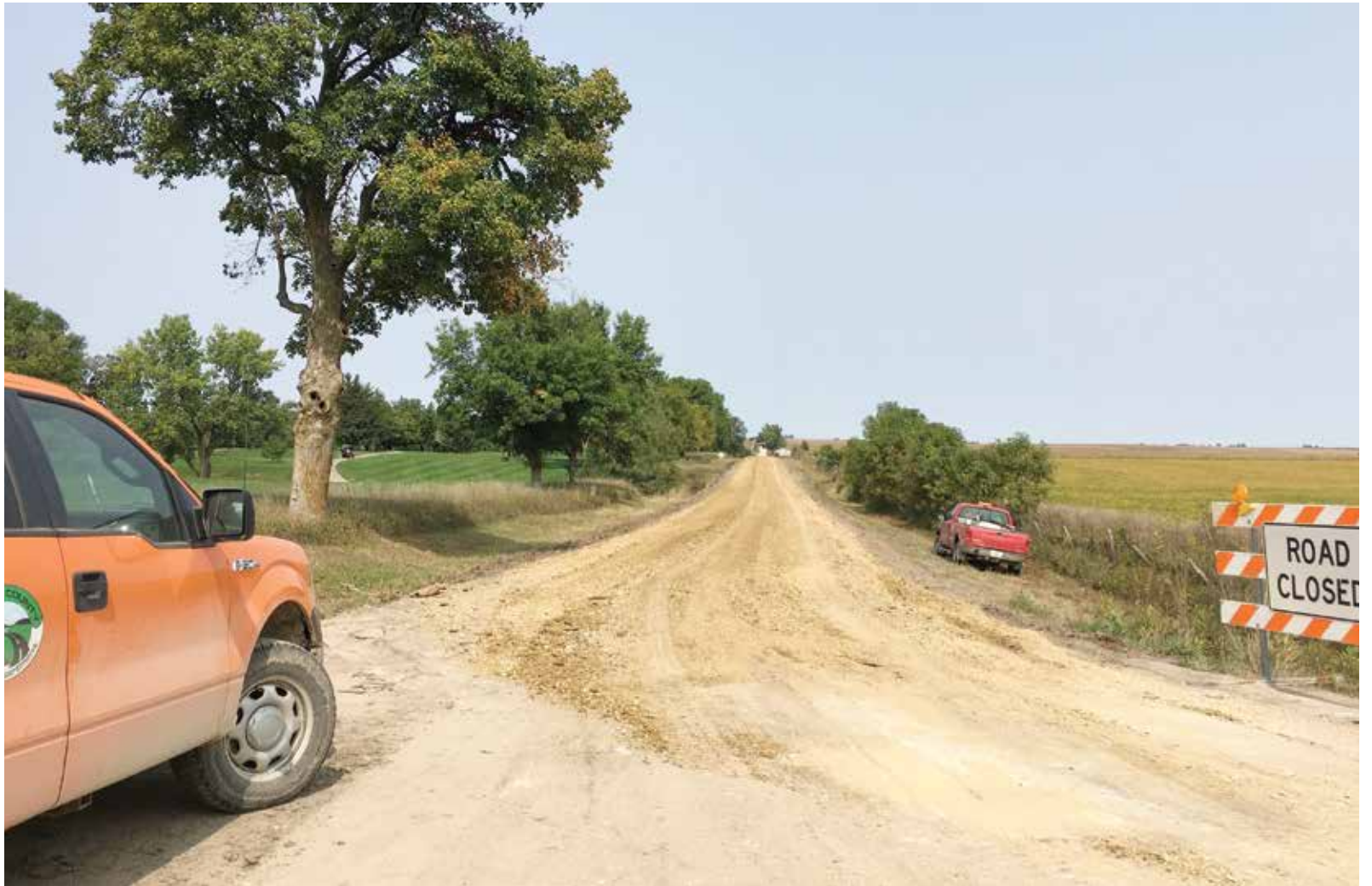
This shows the first section of Sage Trail that was closed for resurfacing, beginning at the corner of 200th Road. Some regrading was done before a 5-inch layer of new material was added to provide something akin to a hard surface, rather than simply gravel, on the road.
