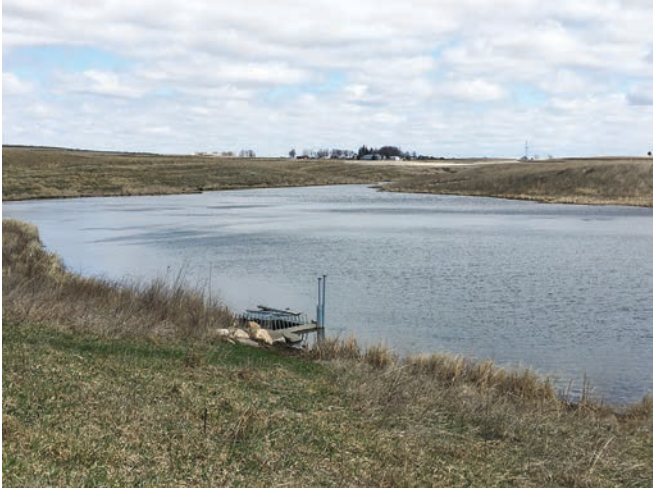
This photo shows the stream entering the wetland near the middle of the far side of the body of water. In the foreground is the outlet that allows water to flow out of the wetland.
