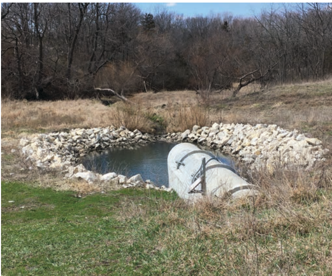
Water from the wetland travels downhill through an underground tube to a splash pool.
