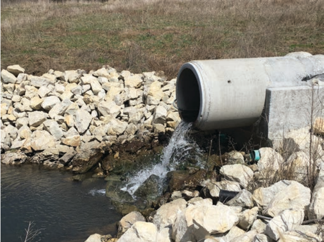
The water coming from the culvert into the splash pool is clear and clean and moves from the pool into a stream on its way to Hughes Cove.
