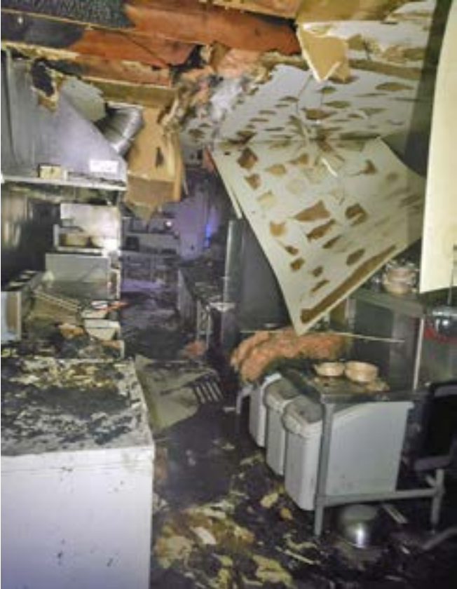
The fire started outside the building, near the kitchen. Flames got into the walls and ceiling of the kitchen, which suffered extensive damage.
