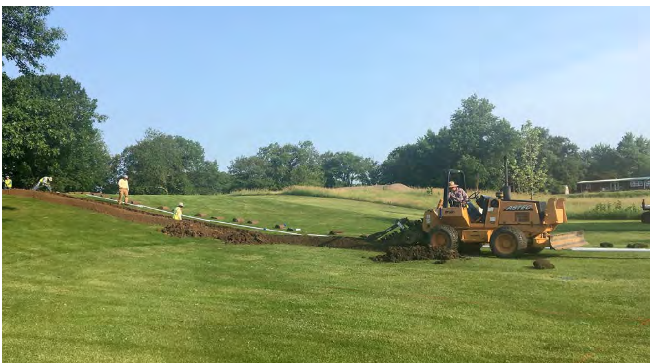
This photo of work underway on the eighth fairway shows the equipment used to dig the trenches for the irrigation lines. Once the lines are placed in the trenches, workers fill the hole and replace sod that was removed.
