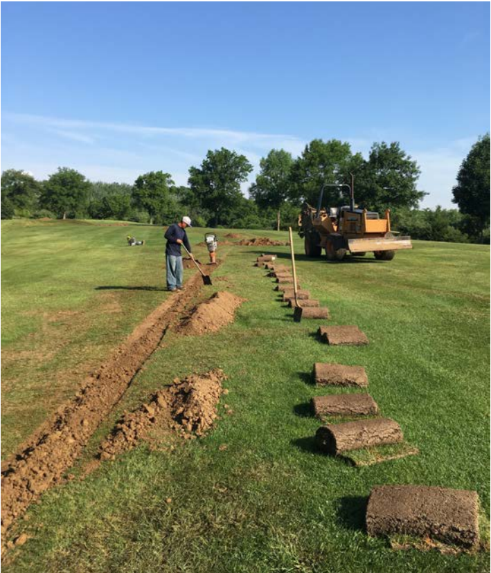
Before the irrigation pipe is trenched in, strips of sod are removed and set aside. Once the pipe is placed in the trench, workers cover it with dirt, then replace the sod.
