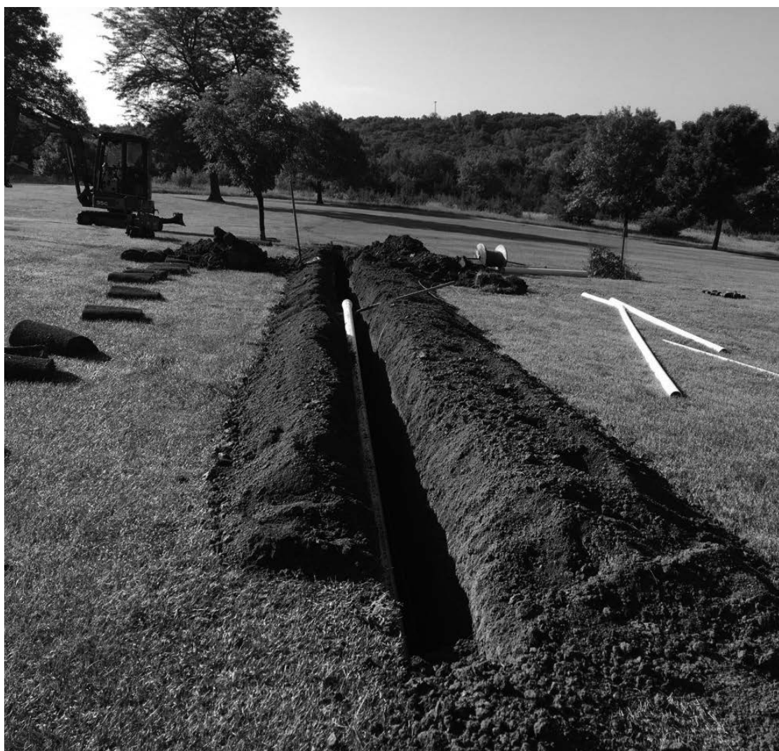
One major project of interest to the LPN greens and grounds committee is the new irrigation system being installed at Panorama West. Work got underway in late May, and involves trenching in pipe to provide water to all tee boxes, fairways and greens on the golf course.
