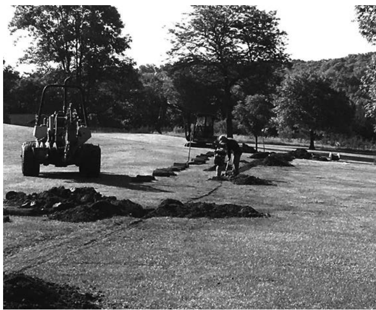
A worker with Landscapes Unlimited uses a shovel and a hand-held machine to tamp down dirt covering a newly installed irrigation line. Rolls of sod are placed on top, which can be seen in the foreground of this picture. The goal is to do as little damage as possible to the existing turf.
