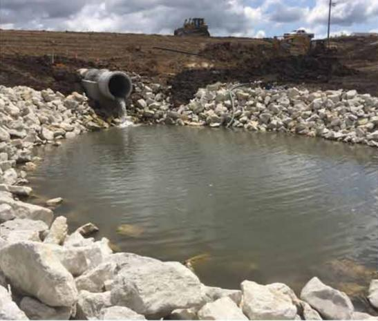
The project consisted of the construction of 23 acres of wetland plus cool season grasses and native grasses. The shallow water wetland includes a control structure above a plunge pool, which routes the water back into a creek leading into Lake Panorama at Hughes Cove. This photo shows the plunge pool.
