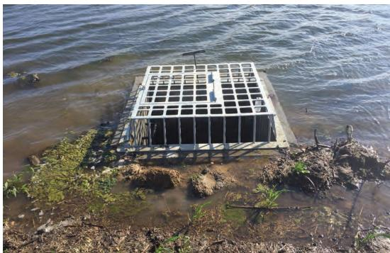
This project is a combination of a dam, sediment filtration area and wildlife habitat. The wetland holds water, trapping nitrogen and other nutrients while also stopping some sediment being carried into the lake. This photo shows the overflow structure at the base of the wetland.
