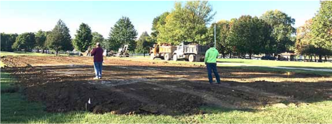
The LPA maintenance staff used a transit to determine how much fill material was needed in various locations. Key components of the prep work were making sure the ground is level, and will drain properly.
