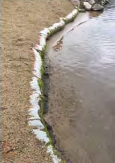
After building a "false floor" for the beach, construction socks filled with recycled tire chips were installed between the water and the beach.
