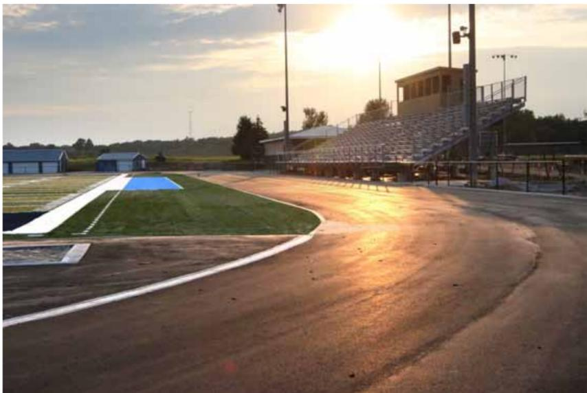
The track asphalt needs to cure 21 days from July 30 before a special coating can be added and the lanes marked.
